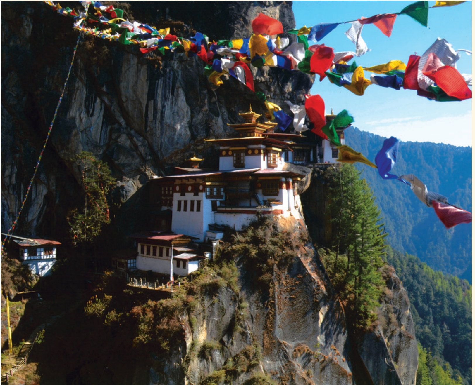
Taksang, popularly known as the Tiger's Lair was damaged by a devastating fire in 1998. His Majesty the Fourth King initiated its rebuilding and the construction was implemented with his blessings. Here we see the rebuilt temples built on top of a cave where Guru Rinpoche meditated in the eighth century after he flew here on the back of a tigress. (Photo: Peter Lowe)
